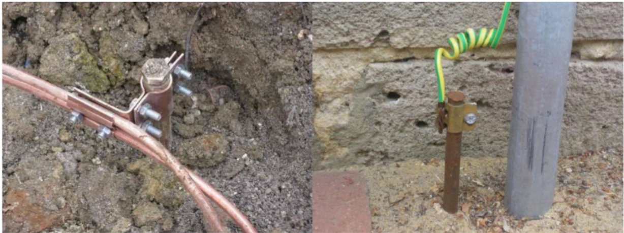
Figure 1: Photographs of grounding applications
